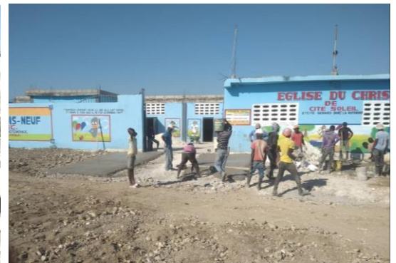
Residents work together to remove the trash, dig a drainage ditch, and pour concrete to make a walkway to the school.
