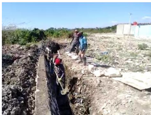
Residents work together to remove the trash, dig a drainage ditch, and pour concrete to make a walkway to the school.
